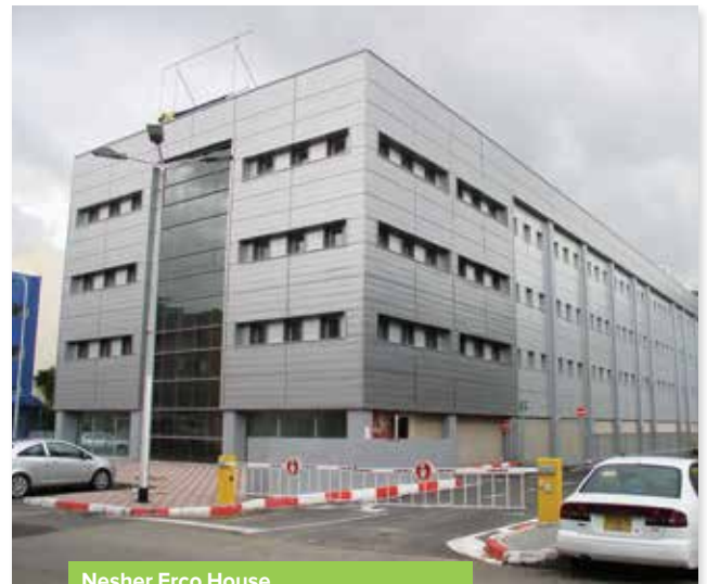
Nesher Erco House, Managed and Maintained by Natam
